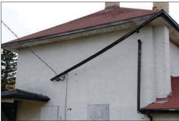
The gutter has fallen off, onto a power line. This is now more than a maintenance issue, but a fire hazard.
