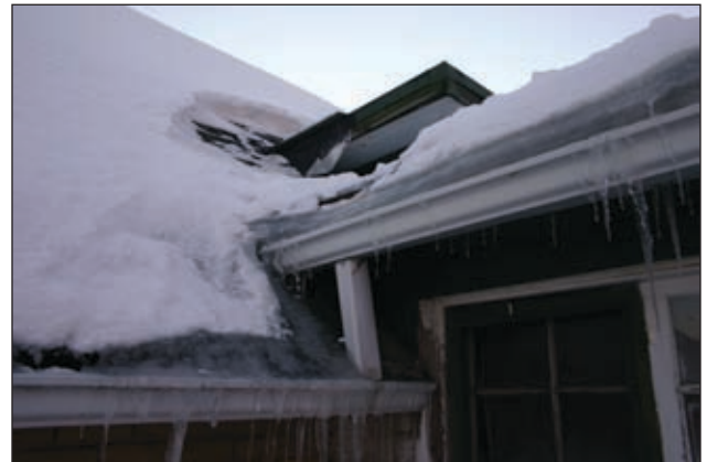
The ice has been allowed to build up at the eaves, potentially damaging the roof line. The best remedy is to improve the insulation in the attic and seal any leaks.
