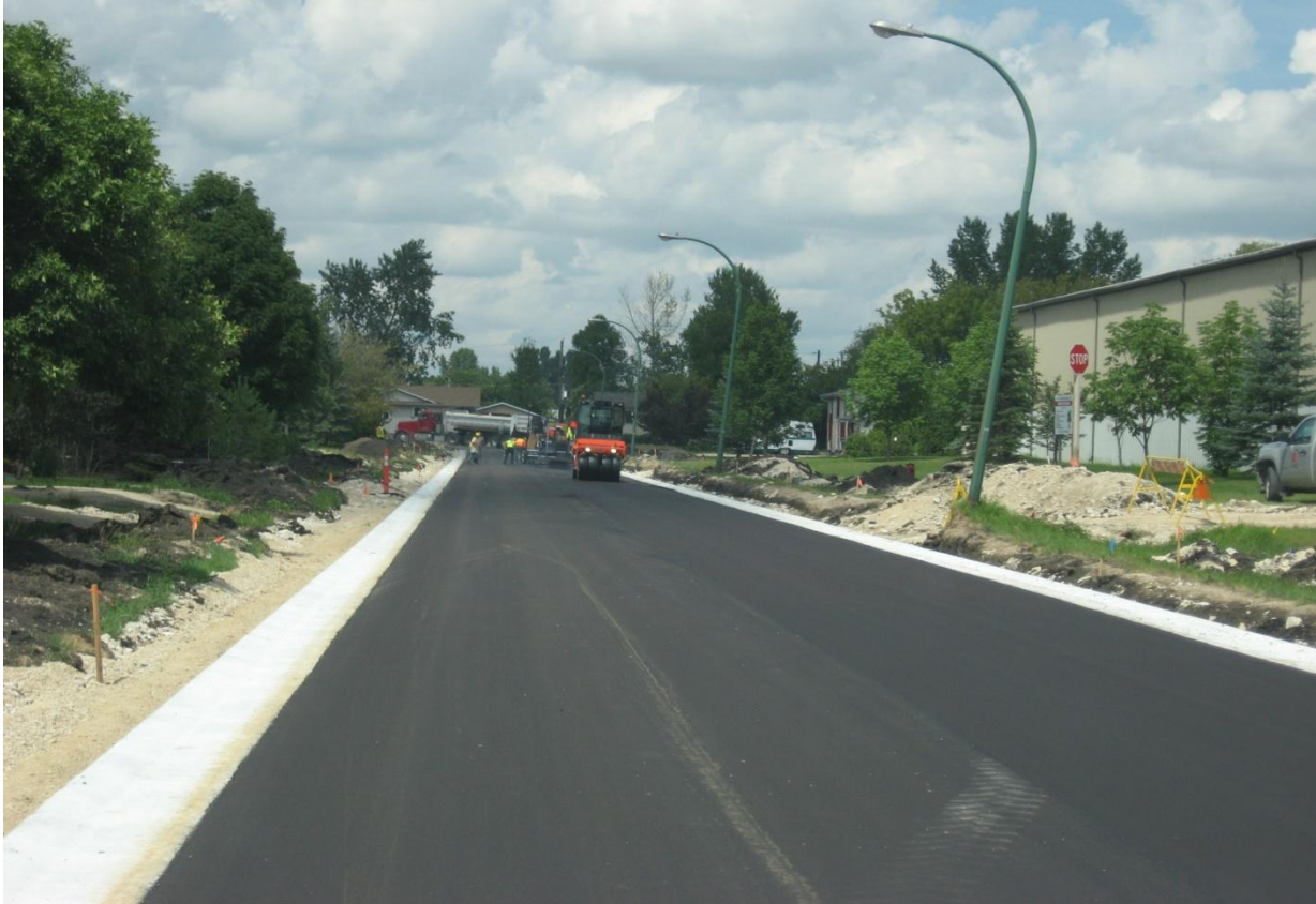
Hebert Road Reconstruction in St. Adolphe
